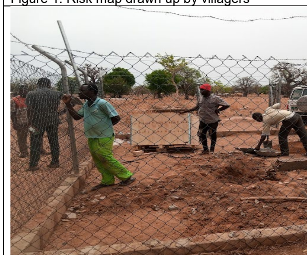
Figure 3: Preparing the ground for meteorological station installation
